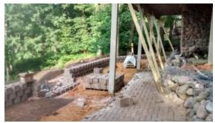
The deck on the home was propped up with temporary bracing, so the contractor could dig out the old pylons and pour new ones. (Photo: Paul's Landscaping)
