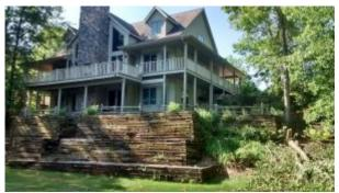
Before: Installed in 1994, this railroad tie retaining wall was in danger of eventual collapse.
