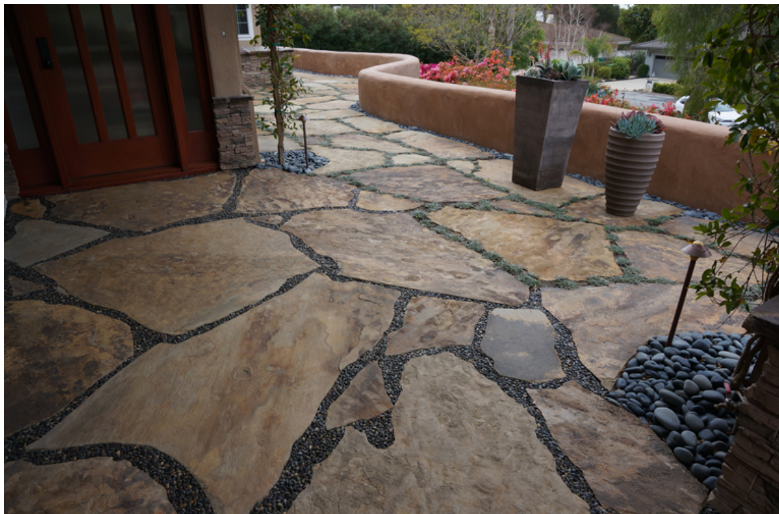
Increased permeability with a flagstone walkway. PHOTO: Wilson Environmental Contracting, Inc.
