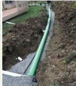
Pictured on the left is an old, failed trench drainage system. To the right is the new system Twin Oaks Landscape installed behind approximately 10 residences in a condominium complex. (Photo: Twin Oaks Landscape)
