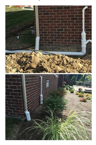
This downspout system avoids drainage problems by tying into a trench drain leading to a retention pond. (Photo: Twin Oaks Landscape)
