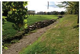
Pictured on the left is a drainage system on a site managed by a homeowners association that had become overgrown and was no longer effective. To the right is a maintained stormwater management solution. (Photo: Twin Oaks Landscape)
