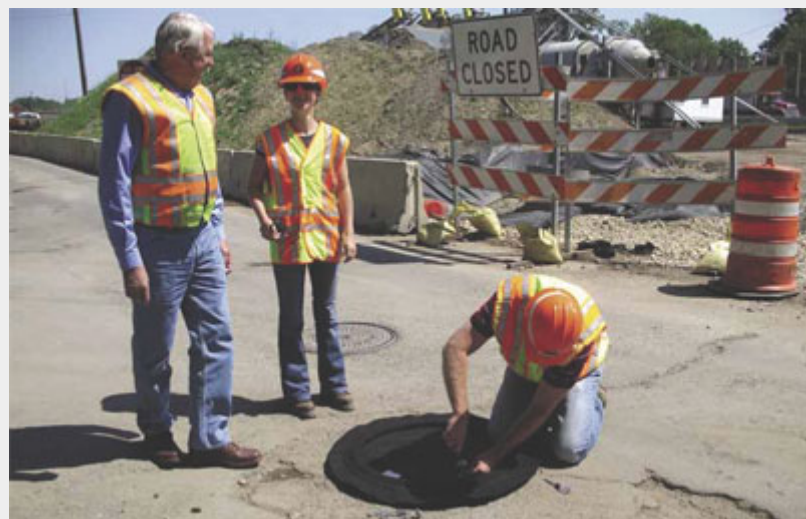
ERTEC’s GR-8 Guard is used on this round grate to reduce sedimentation. Lawn and Driveway is a distributor for the company.
