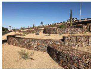
Gabion baskets are typically used near slopes and banks to combat water erosion.
